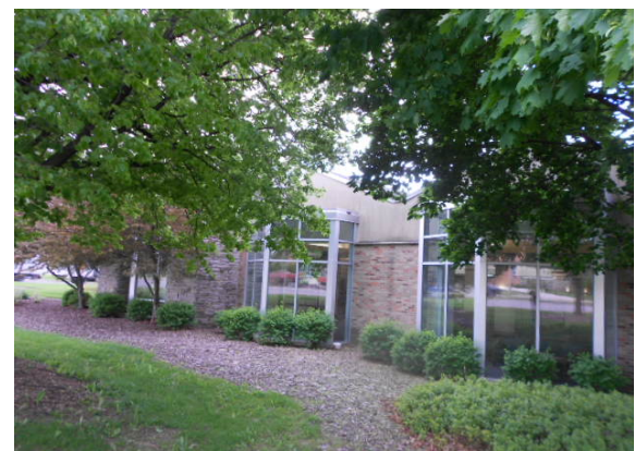
Photo #30: Exterior Insulation and Finish System (EIFS) North elevation (east end)
