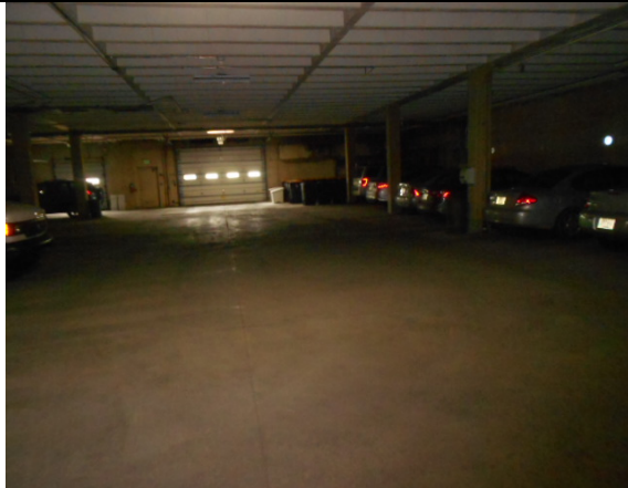
Photo #23: Subterranean parking garage
