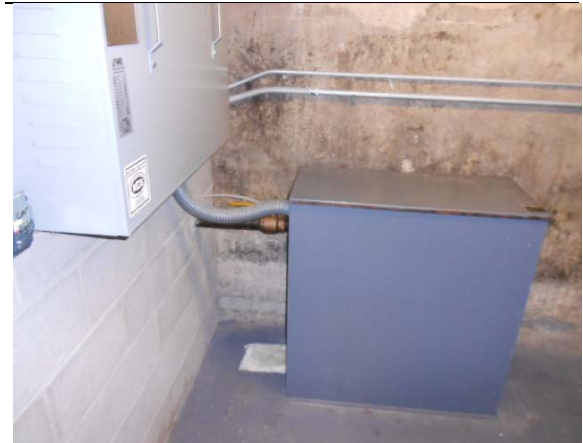
Photo #50: Elevator equipment
