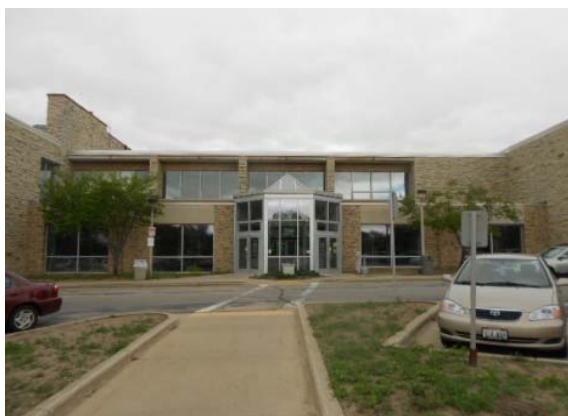
Photo #5: Rear (south) elevation at main entrance
