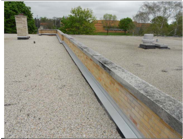
Photo #28: Parapet wall between City Hall and Civic Center
