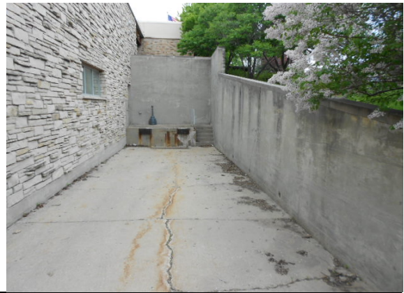
Photo #16: Retaining wall at loading dock at Library
