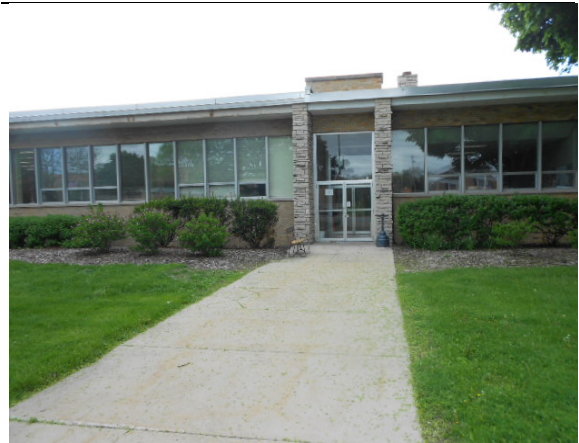
Photo #32: Windows and entrance doors
