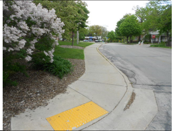
Photo #10: Concrete sidewalk and curb cut
