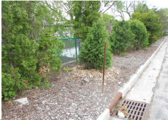
Photo #19: Site fencing
