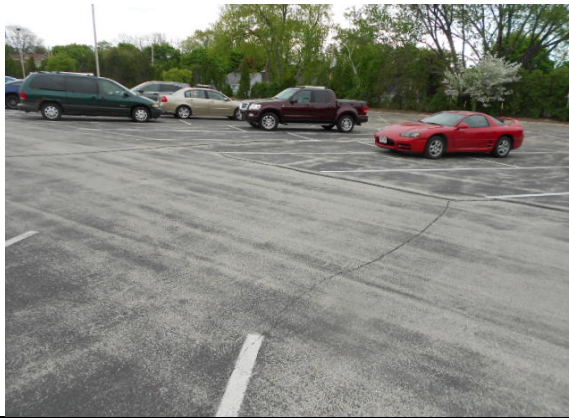
Photo #9: Asphalt pavement at parking lot
