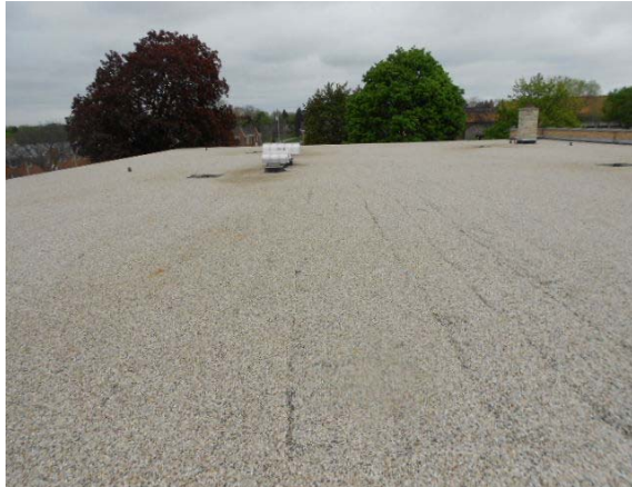
Photo #7: Roofing – modified bituminous membrane
