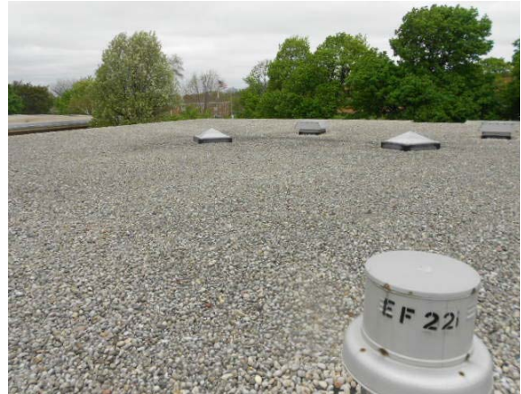
Photo #8: Roofing – EPDM membrane with stone ballast
