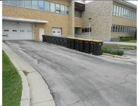
Photo #34: Overhead door to subterranean parking garage
