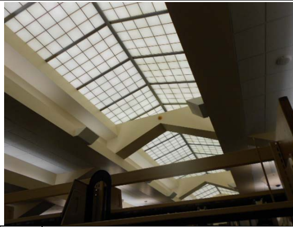
Photo #27: Skylight at Library
