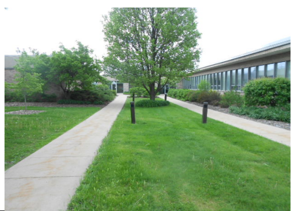
Photo #18: Walkway lighting
