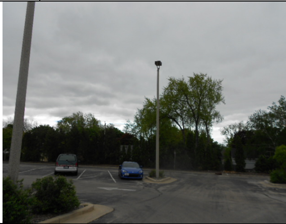
Photo #15: Site lighting
