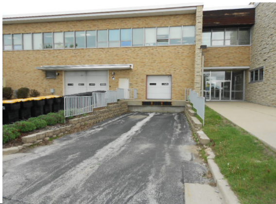
Photo #17: Retaining wall at loading dock at City Hall
