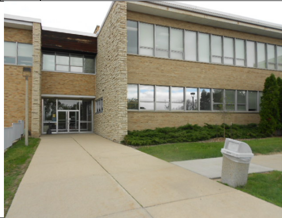
Photo #33: Windows and entrance doors
