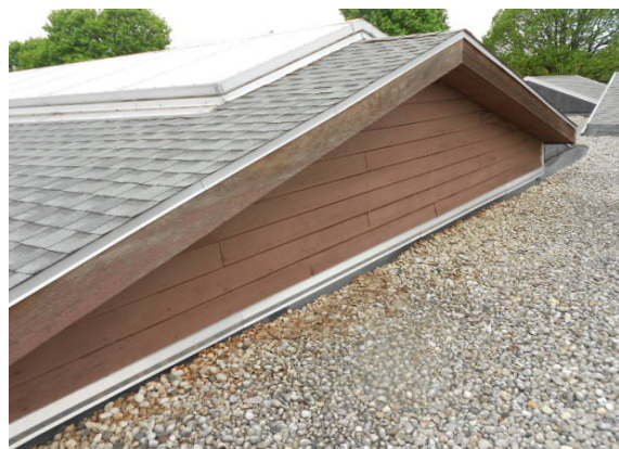
Photo #29: Wood siding and trim
