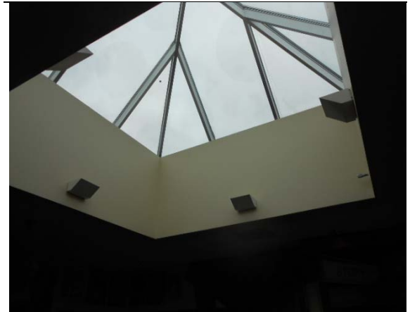
Photo #26: Skylight at Library
