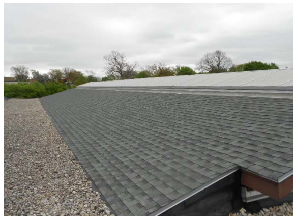
Photo #24: Asphalt shingle roofing
