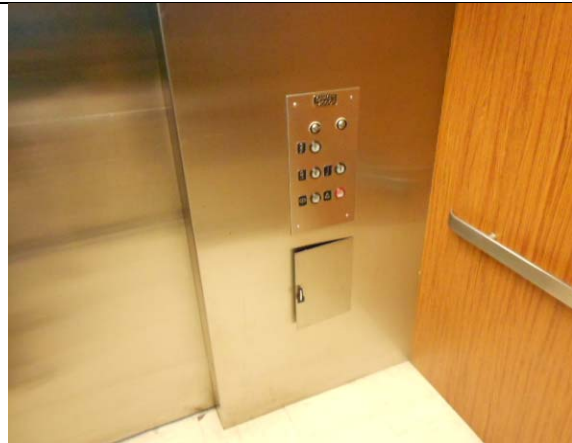
Photo #49: Elevator cab interior
