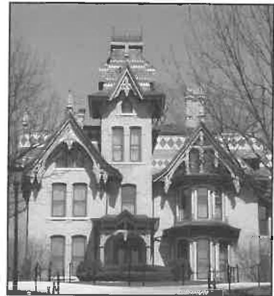
Appropriate: Color creating pattern in unexpected materials; the roofing establishes the color scheme on this historic home (8000 Milwaukee Street).
