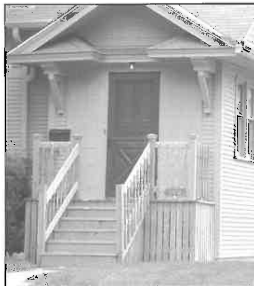
Inappropriate: Unpainted pressure treated wood without period detailing already evident on building.
