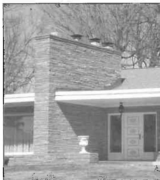
Large, projecting, lannon stone chimney (7230 W. Wells Street).
