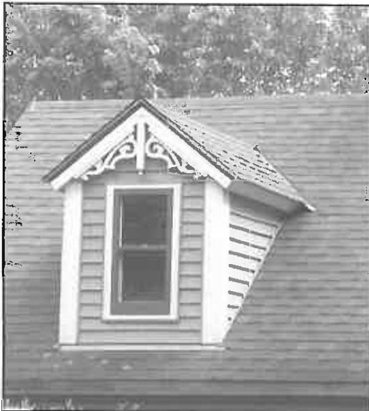
Ornate bargeboard on dormer (1412 St. George Street).
