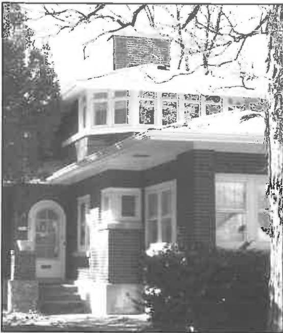
Classic Prairie style forms: wide overhanging eaves, central chimney element, bands of windows, intersecting hipped roofs (7917 Stickney Street).
