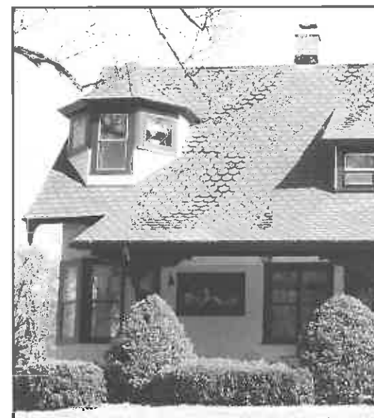
Corner turret with leaded glass windows, scalloped-shaped roof shingles (8028 Warren Avenue).
