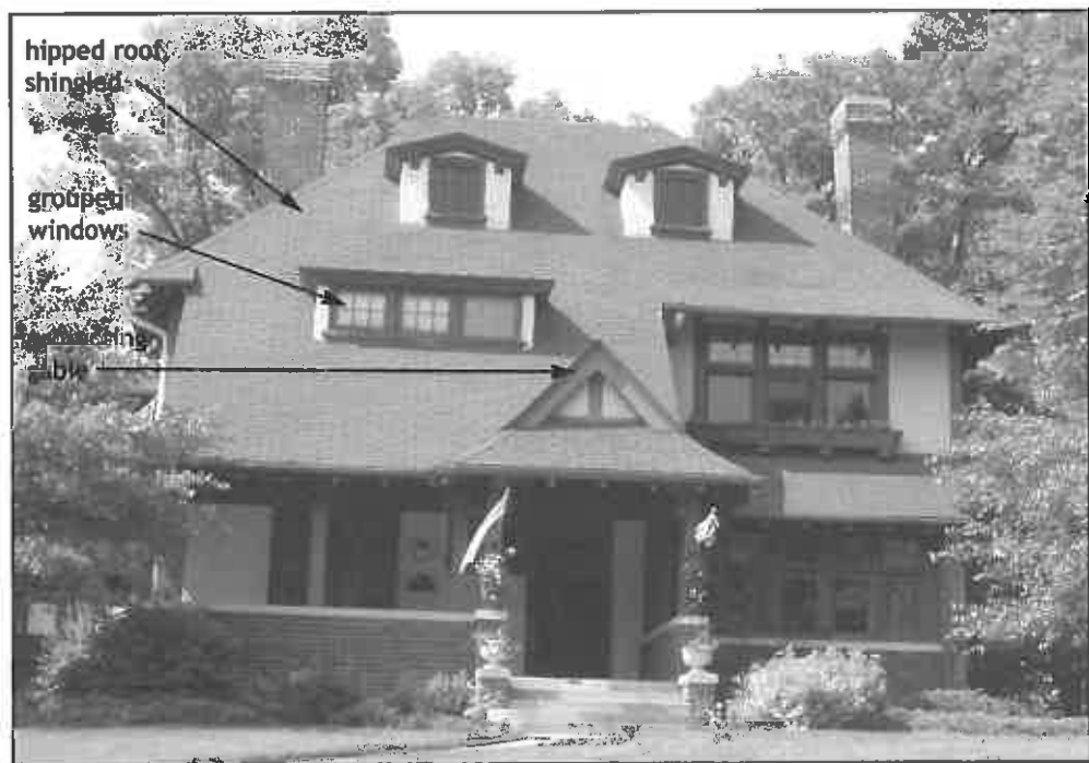
Craftsman home with multiple dormers and a long, low porch (7424 Kenwood Avenue).
