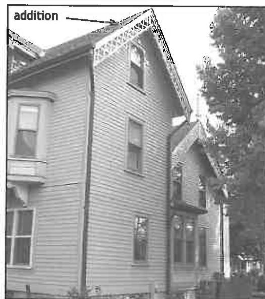
Appropriate Rear Elevation Addition: This substantial addition does not interrupt the scale, massing and character of the existing home. The detailing and materials of this addition are similar to that of the existing home, without being exact copies. (1609 Church Street).
