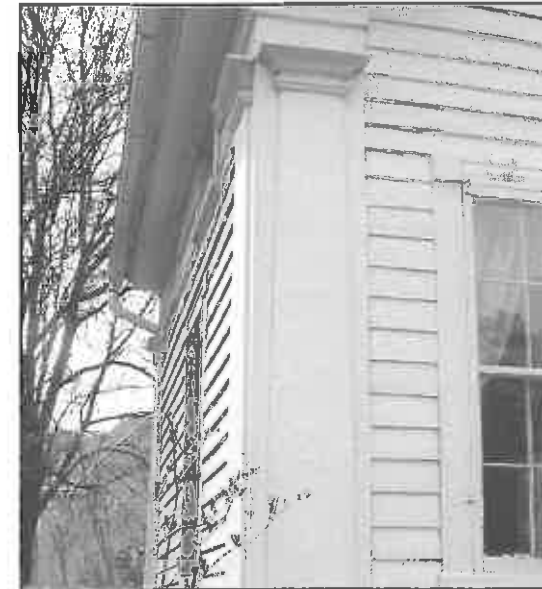
Simplified pilaster (2107 N. Wauwatosa Avenue).
