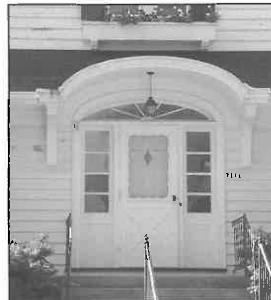
Side-light windows flanking door, topped with a fan-light (7111 Maple Terrace).
