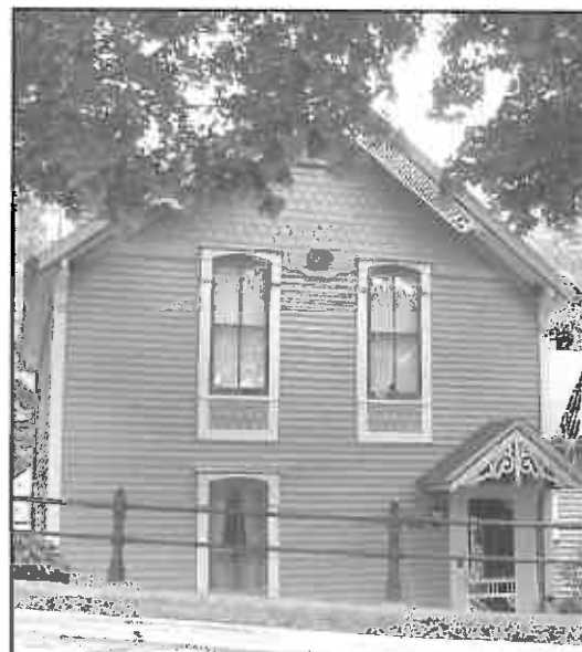
Gothic Revival home (1412 St. George Street).
