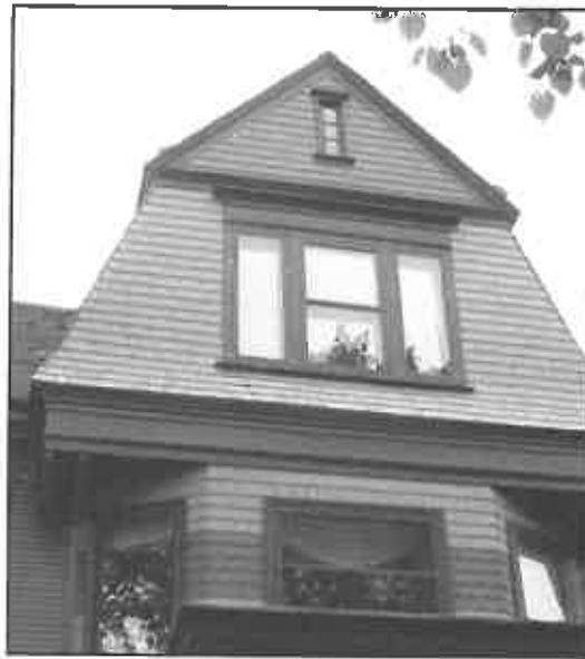
Appropriate: Color used to highlight change in shingle profile and detailing (7406 Hillcrest Avenue).
