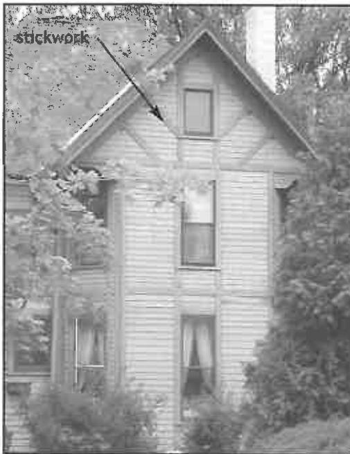
Stickwork in gable end (1735 Church Street).
