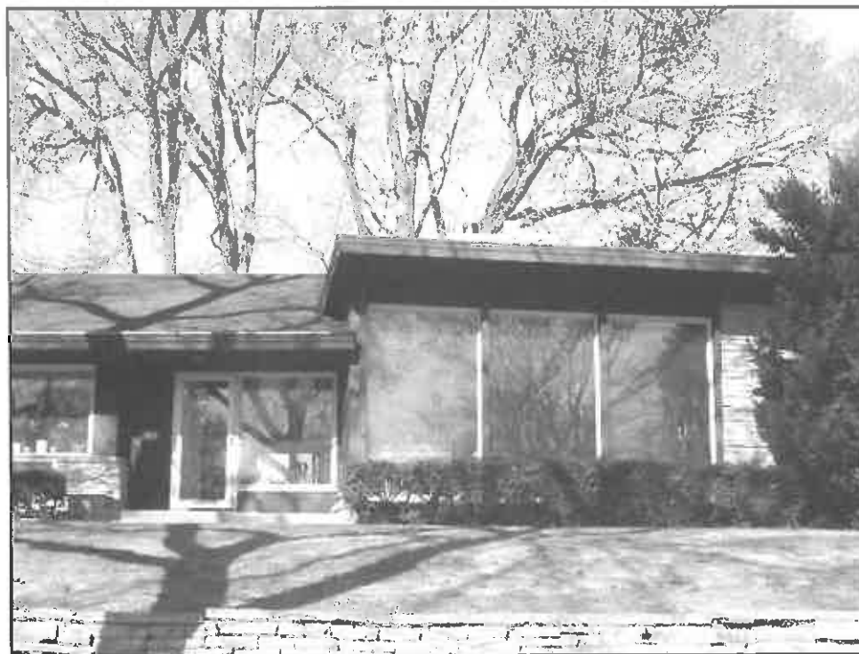
Flat roof & large plate glass windows on Contemporary home (6564 Washington Circle).
