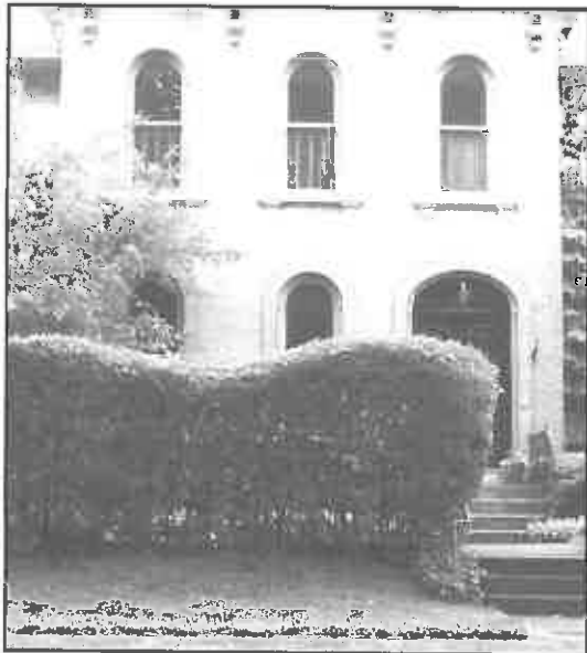
Inappropriate: Scale of shrubs is too tall & informal for the symmetrical Italianate style home.
