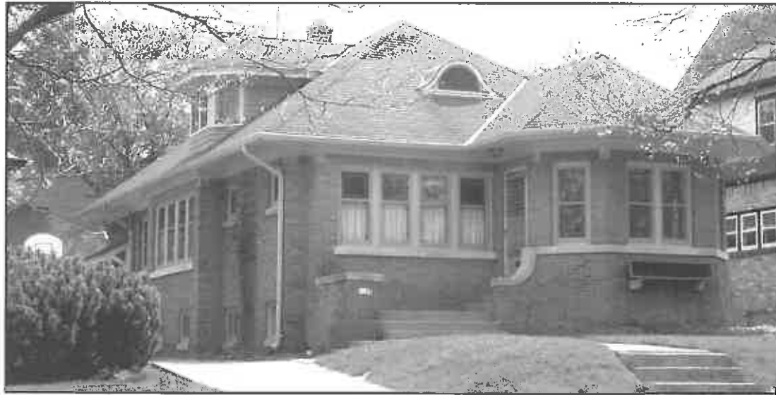
Bungalow home with projecting bays and eyebrow window (6619 W. Lloyd Street).
