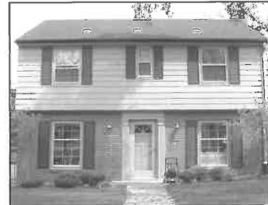
Two-story Minimal Traditional home, second floor walls project slightly beyond the first floor evoking a Colonial detail (1804 Alta Vista Court).
