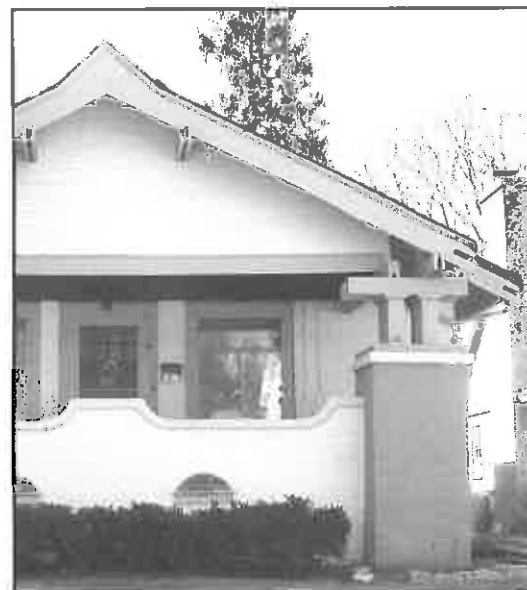
Crafted joints and cutouts on wood beam and rafter ends (8011 Stickney Street).
