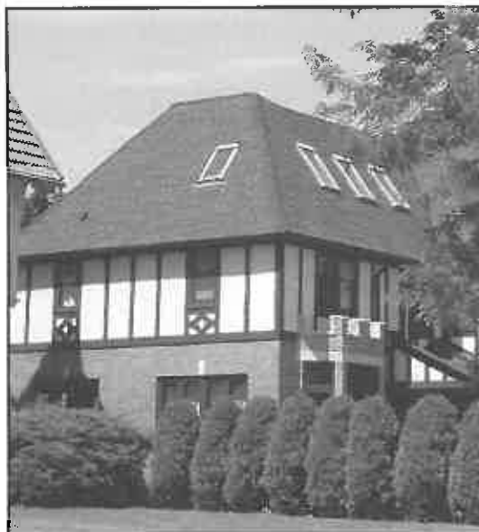
Inappropriate: Skylights placed prominently on the front and side elevation of the home disrupt the roofline.
