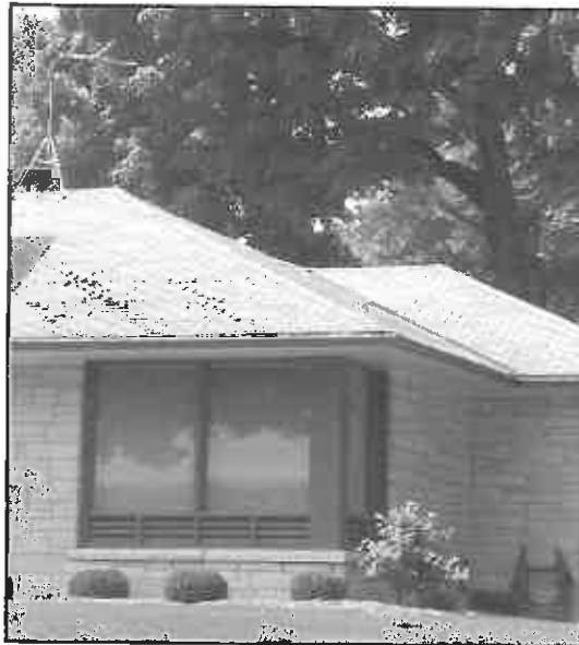
Large corner picture window with louvered vents below (7208 Wells Street).
