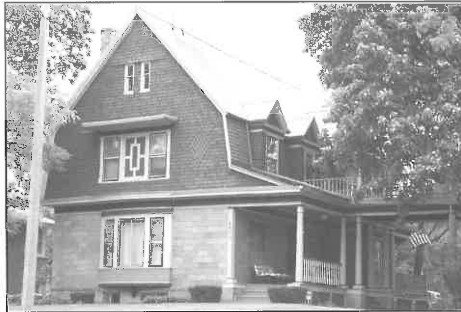
Side gambrel roof on an ornate Dutch Colonial home (6200 W. Wisconsin Avenue).
