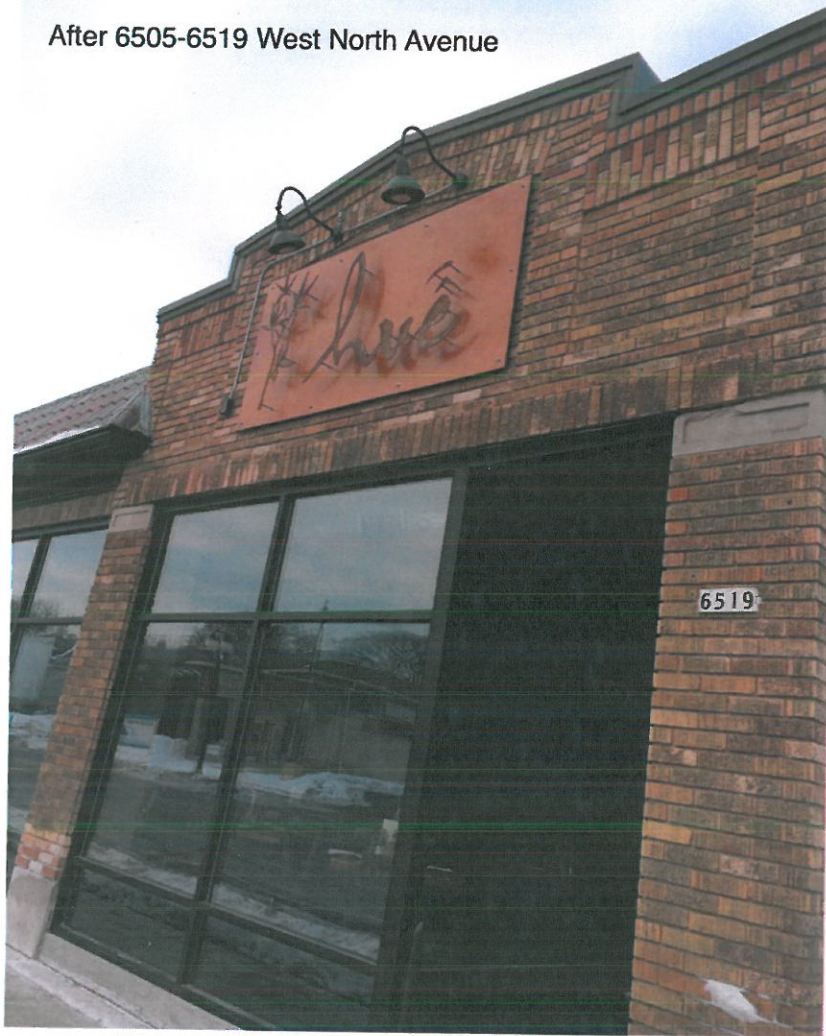
After 6505-6519 West North Avenue Hue Patio Space
