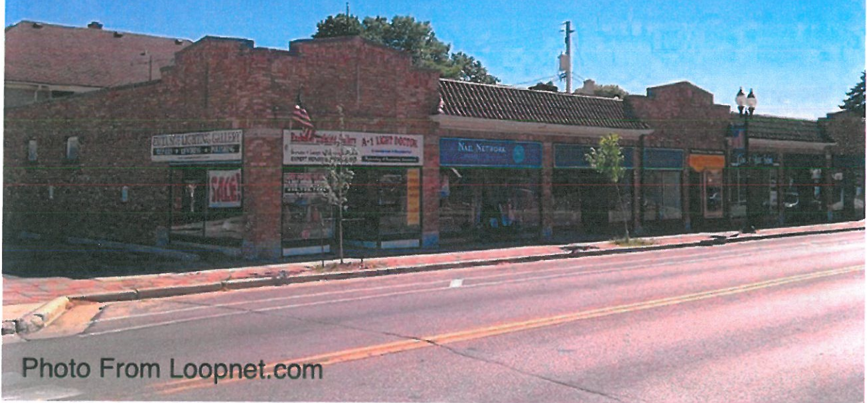
Before 6505-6519 West North Avenue
