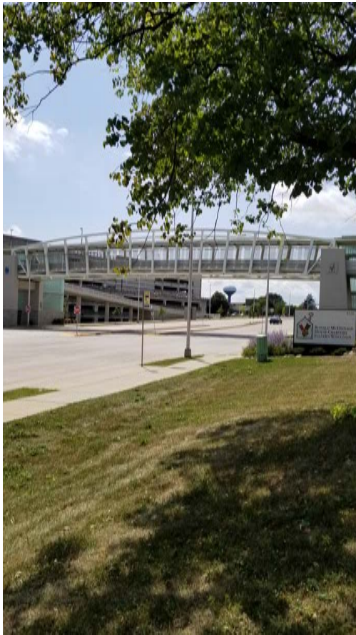
Watertown Plank Road pedestrian bridge
