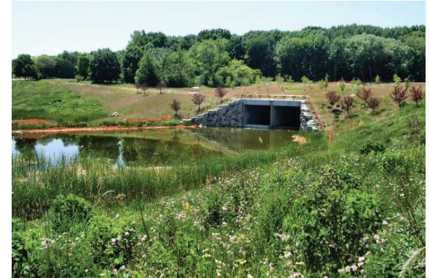
The MMSD Flood Management Basins serve the primary role of flood risk mitigation, while also creating vistas of the area's abundant natural features. Source: MMSD
