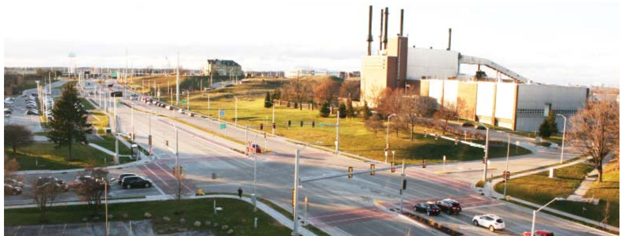
Watertown Plank Road looking west at 92nd Street. Source: GRAEF
