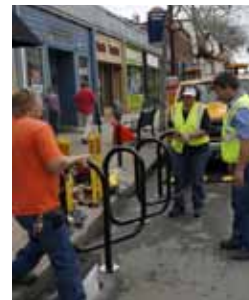
Bike Corrals. This technique converts an on-street parking stall to bicycle use on a seasonal or permanent basis.
