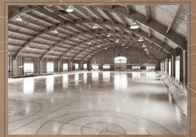
Photo courtesy of Sentinel Structures, Inc.
