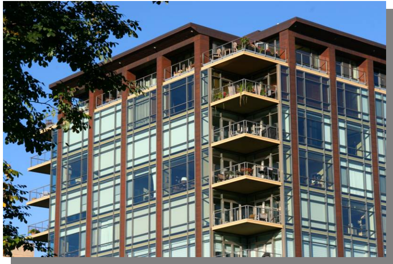
Example of Urban Density Multi-Family: Extensive use of glass and brick, an articulated façade, and balconies
