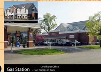
F Gas Station - 2nd Floor Office - Fuel Pumps in Back
