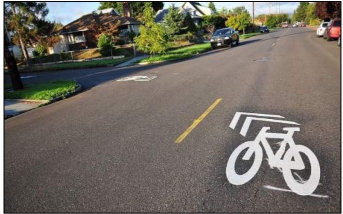
Figure 5: The chevrons on a SLM can be angled to indicate a turn in the route as shown in this example from Portland, OR, which may require FHWA experimentation.
