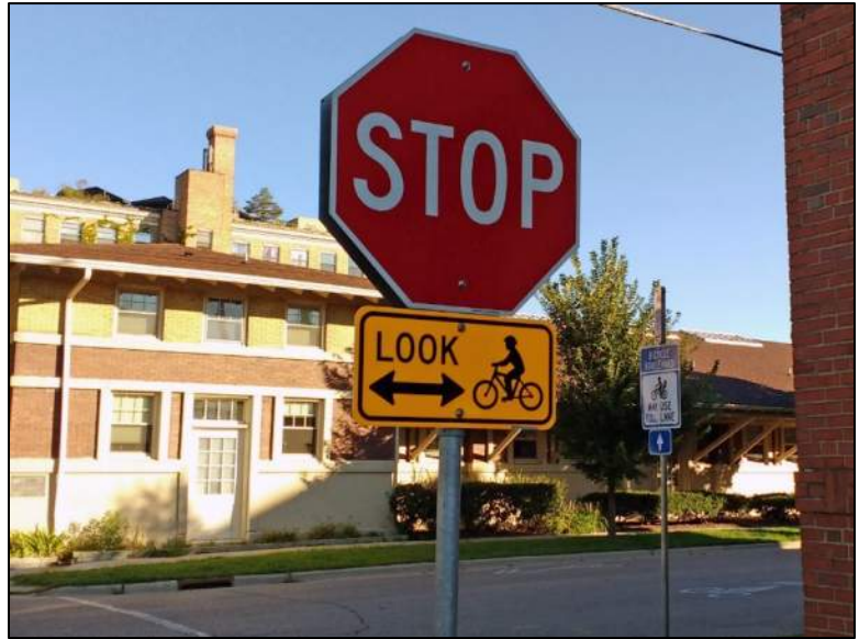
Figure 19: Example of a supplementary sign warning people to look for bicycle traffic at a location where the stop control was "flipped" from the neighborhood greenway to the local cross street.
