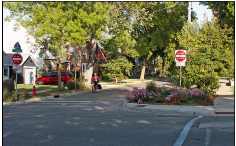
Figure 18: Example of a curb extension used as a traffic diverter on the Kendall Avenue Bicycle Boulevard in Madison, WI. The curb extension allows space for bicyclists to enter the street, but a DO NOT ENTER sign prohibits vehicular traffic.
