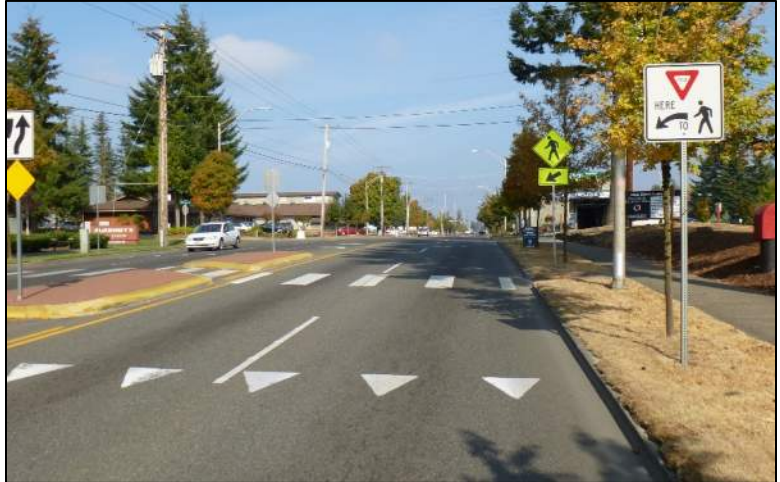
Figure 22: Example of a pedestrian refuge island combined with high visibility crosswalk markings, an advance yield line, and crossing warning signs
