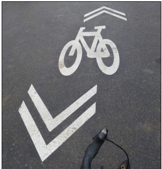
Figure 6: Example of a bi-directional SLM, which may require FHWA experimentation.
