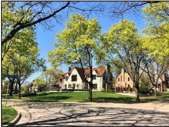
Intersection of Brookside Place and Rockway Place
