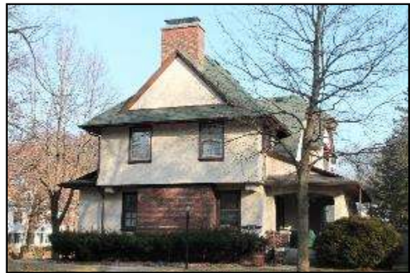
House, 1910 836 N. 67th Street
