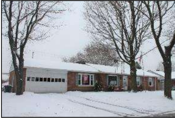
William H. Cox House, 1951 556 N. 105th Street
