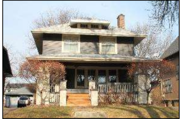
House, 1910 6912 Cedar Street
