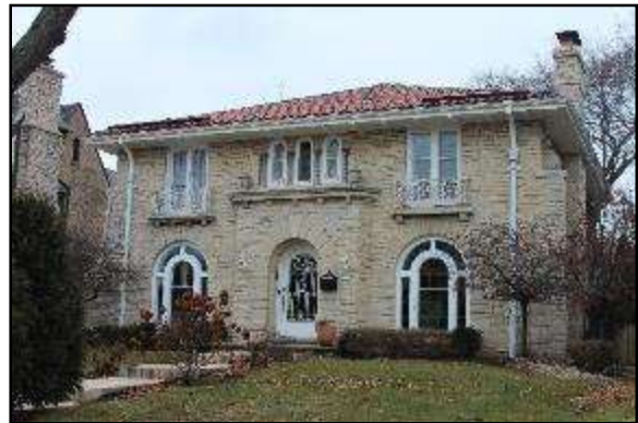
Frances Seefeld House, 1930 7237 Wisconsin Avenue
