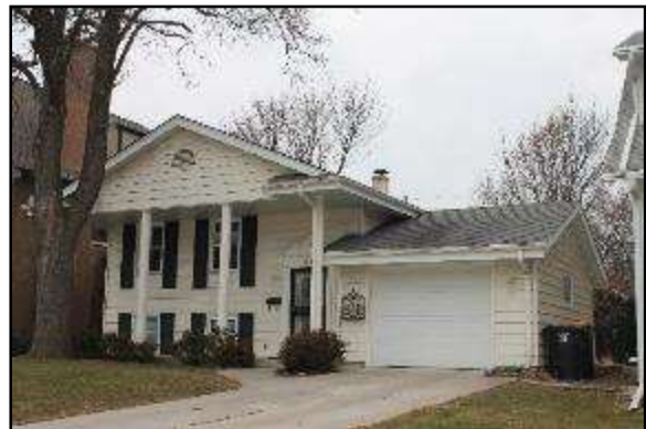
Helmuth O. Knorre House, 1971 7124 Wisconsin Avenue
