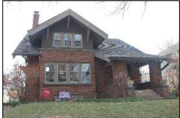
House, 1914 6913 Cedar Street
