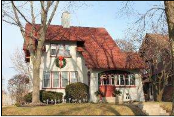
House, 1916 6934 Cedar Street
