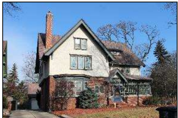
House, 1908 6726 Cedar Street
