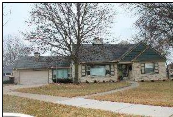
Robert Rasmussen House, 1950 7515 Wisconsin Avenue
