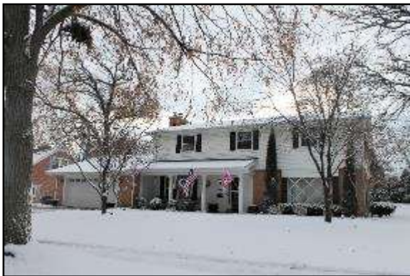
Albert Little House, 1965 7033 Wellauer Drive
