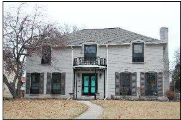
Mowat Waldren Jr. House, 1965 7704 Wisconsin Avenue
