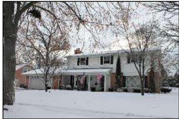
Albert Little House, 1965 7033 Wellauer Drive
