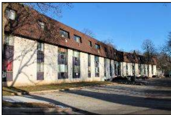
Tosa Glen Apartments, 1977 1330 St. James Street
