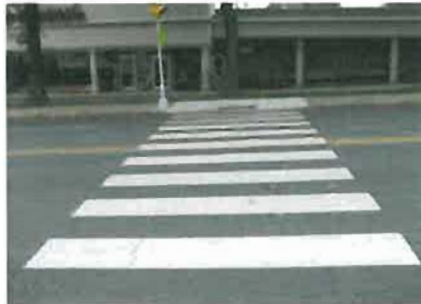
Figure 25: High-Visibility 'Continental' Crosswalk
